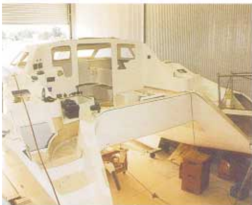
ABOVE: A Lightwave under construction.
